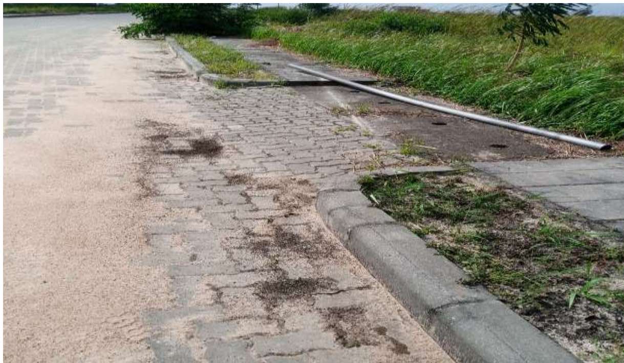
Figure 2: Architectural adaptation strategy (permeable road pavement, green verge by the road, and covered drainages to prevent indiscriminate refuse disposal) Source: (Researcher, 2024)
